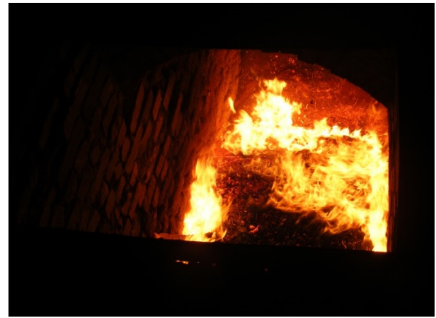
Fig. 2. Use of primary wood waste to obtain heating energy: 1 – waste before loading to the boiler, 2 – burning waste in the boiler.
